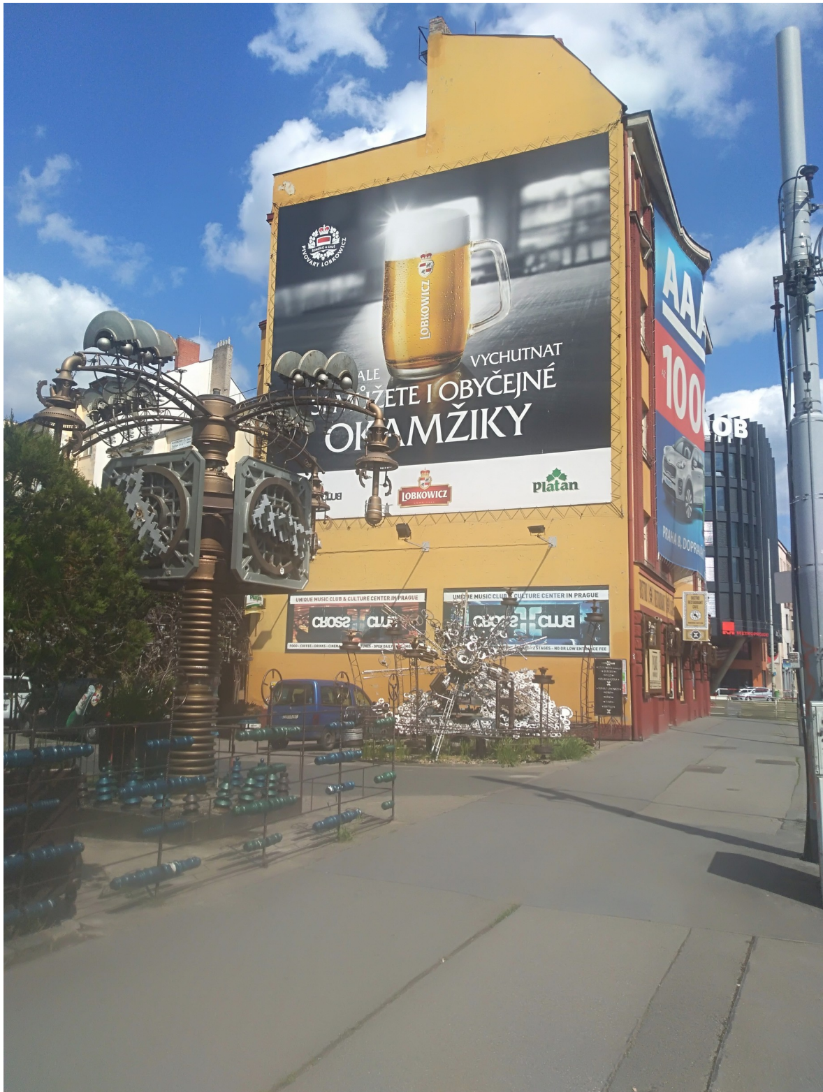
Figure 4: The building housing Cross club from the direction of Nádraží Holešovice. Photo by author. 2020. It is possible to see the advertisement on the building, as well as unique metallic statues that are part of the venue's design. The metallic scaffolding is situated on the left side of the building.
