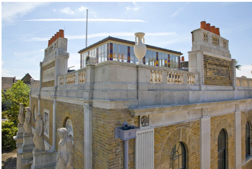
68. John Soane, Pitzhanger Manor – lucerna exteriér, 1801–1804
