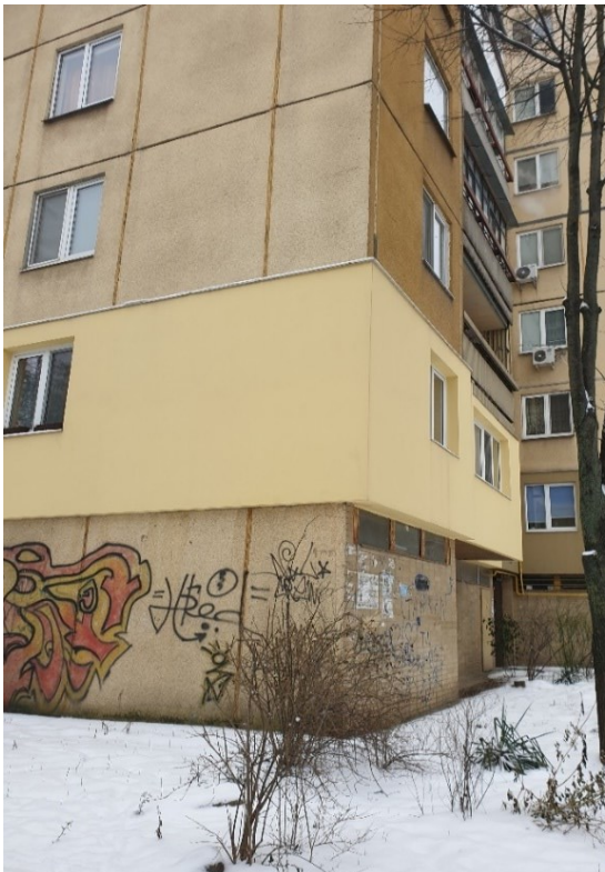
Figure 3.5.: Wall insulation in multi-family homes, Uzhhorod, Ukraine.
