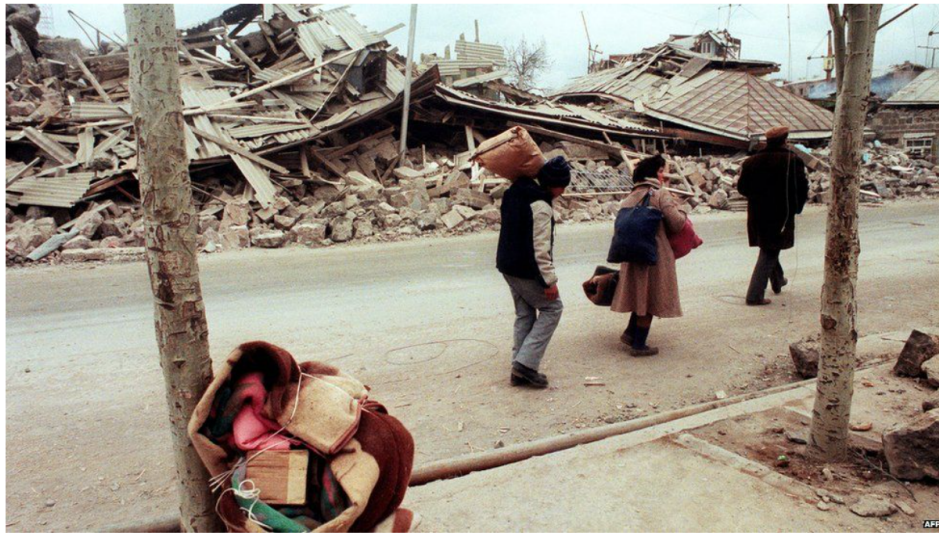
Figure 3.B3: Note: This picture illustrates episodes from the 1988 Armenian Earthquake.
