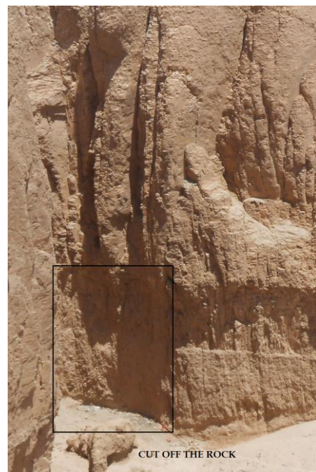
Fig.II.9 – Cut off the rock (photo author)
