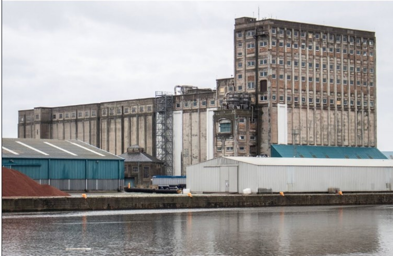
7. Silo, Leith, Edinburgh, 1933
