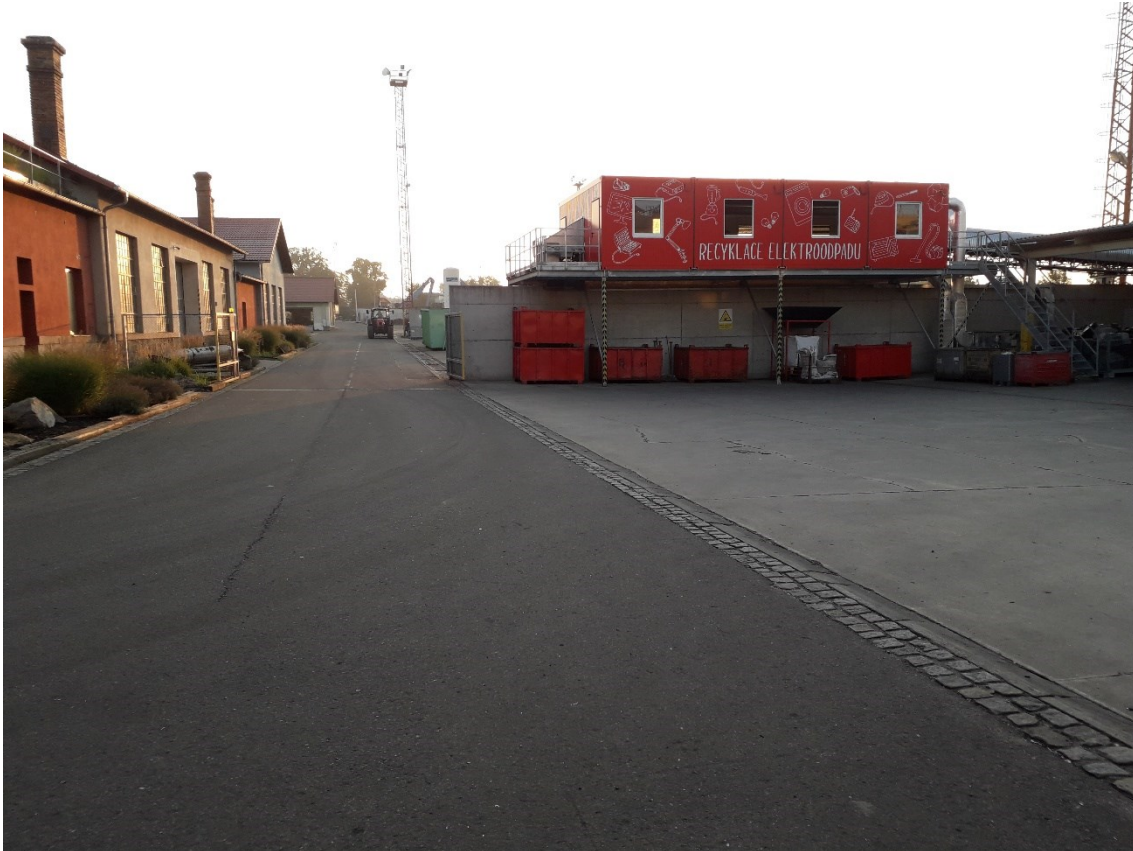
Figure 9 The portable building
