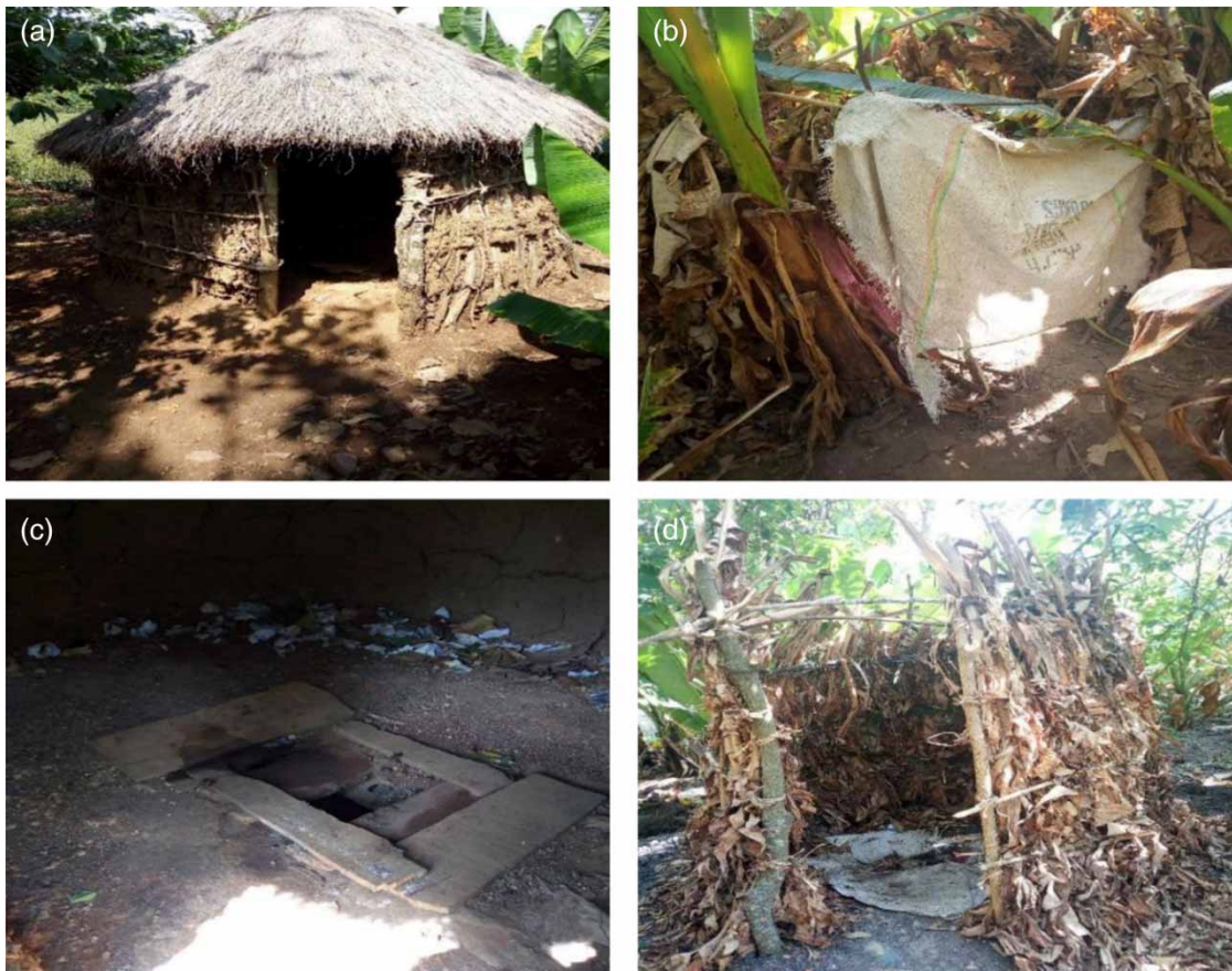
Figure 2 | Examples of latrines in the study area. Notes: Pictures A and C show an improved pit latrine with a roof, solid walls, and a solid plastered slab platform, respectively. Pictures B and D are the examples of low-quality nondurable latrines typical for the study area.
