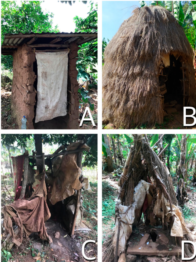
Figure 5. Examples of sanitation facilities. A – a pit latrine with a tin roof, a solid slab and water for handwashing. B – a pit latrine with a grass roof and a solid slab. C and D – Collapsed tin and grass roof latrines with solid slabs but without solid superstructures. Both still in use.
