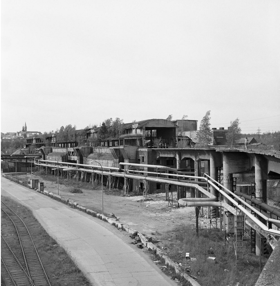
Img. 41 A view from the bridge towards the derelict iron ore storage, 2009, photo by author
