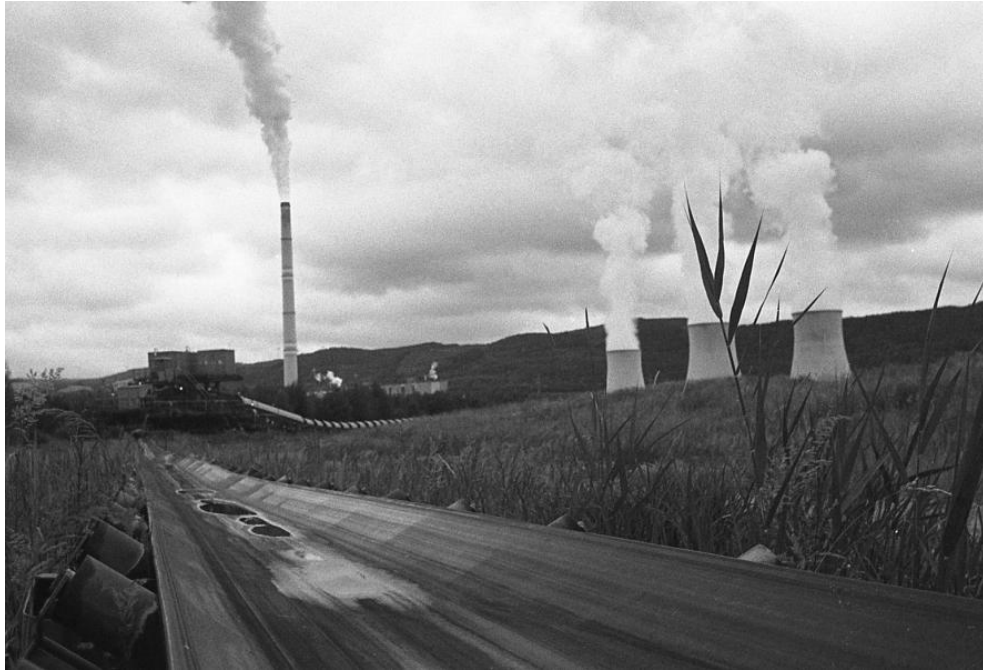
Img. 79 Belt conveyor in the rehabilitated land, 2011, photo by author
